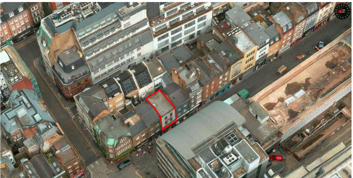
Satellite view over Berwick Street towards Duck Lane
