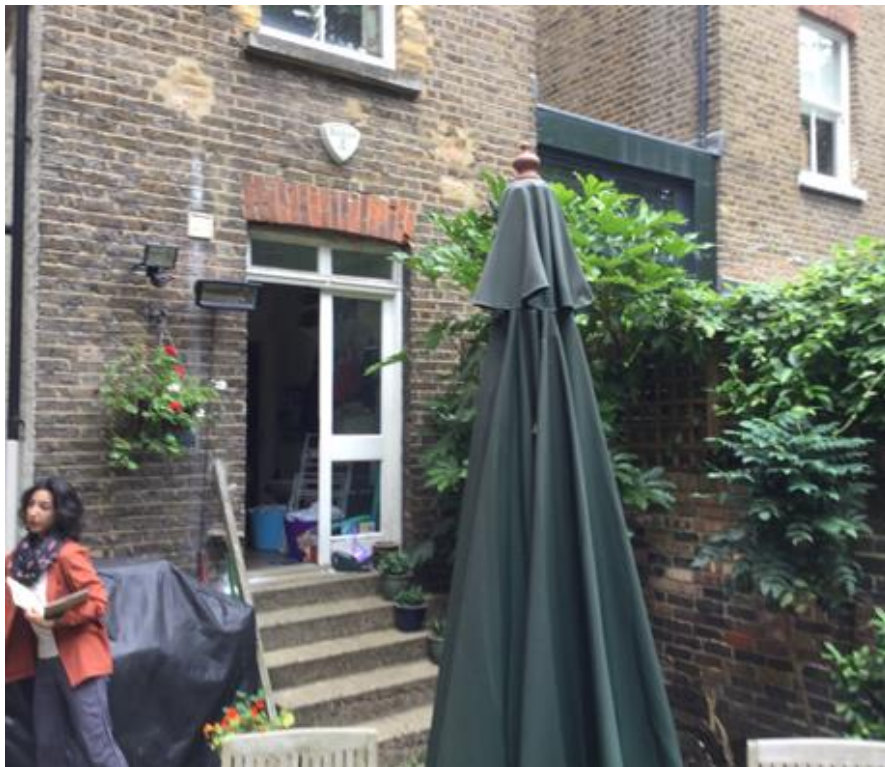
View of existing closet wing
